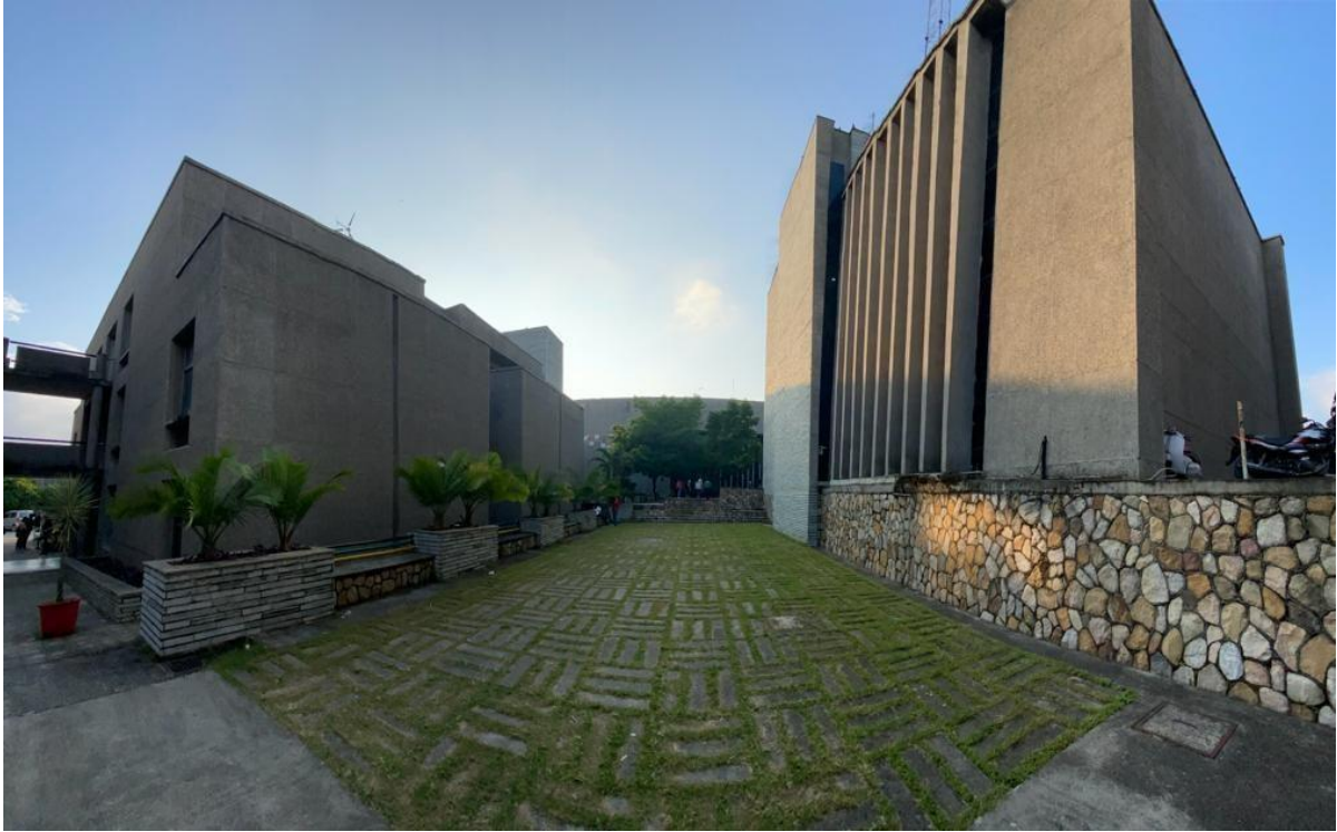
Figure 5 Architectural elements used to combat with the climate along with the use of rubble masonry that can also be seen also the in between spaces were designed in an interesting manner with the use of grass cell pavers.
