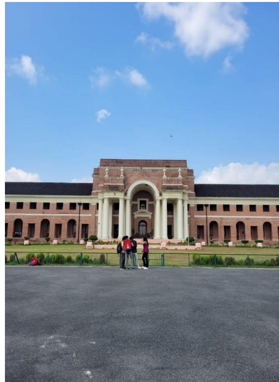
Figure 4 A view from road leading inside the campus
