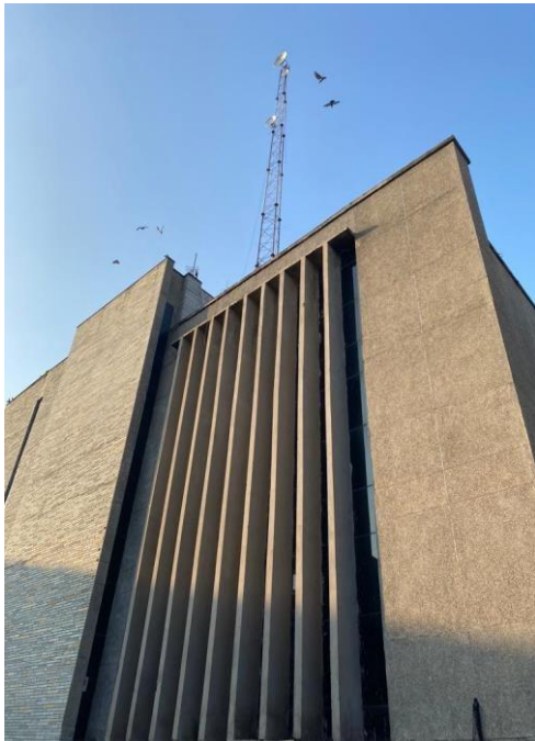
Figure 3 Fins and recessed glass windows used
