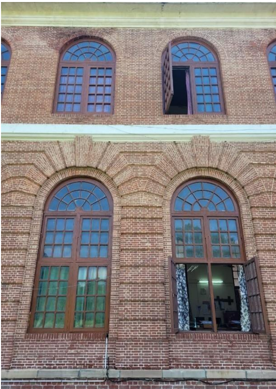
Figure 3 Exterior facade with arched windows
