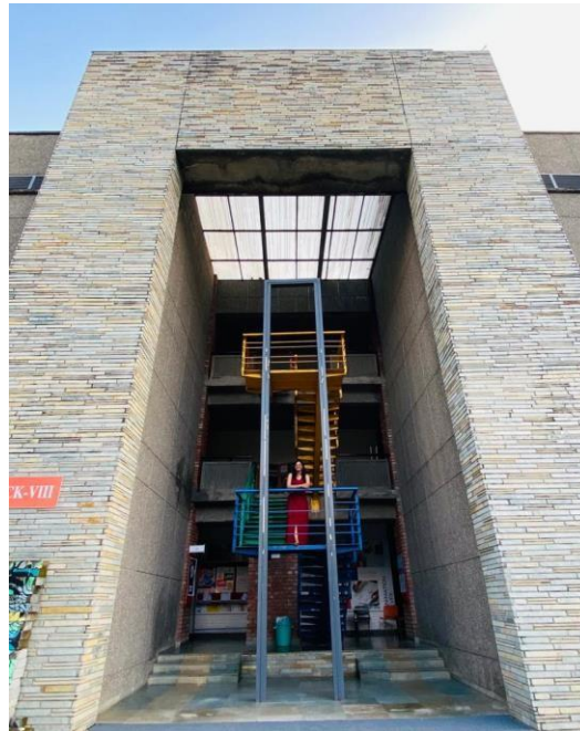
Figure 4 Thin slabs of Kota stone used on the facade
